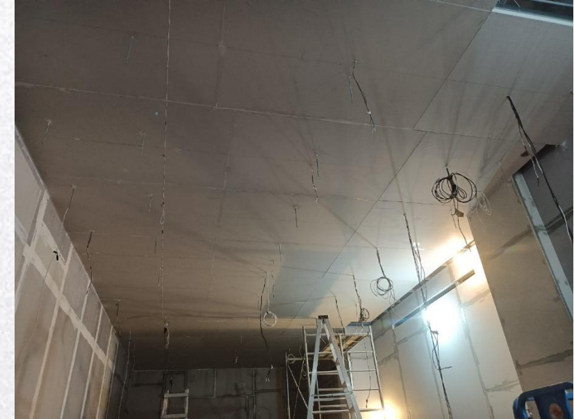
2.3cm Thick Complex Sound Insulation Panels (after construction)
