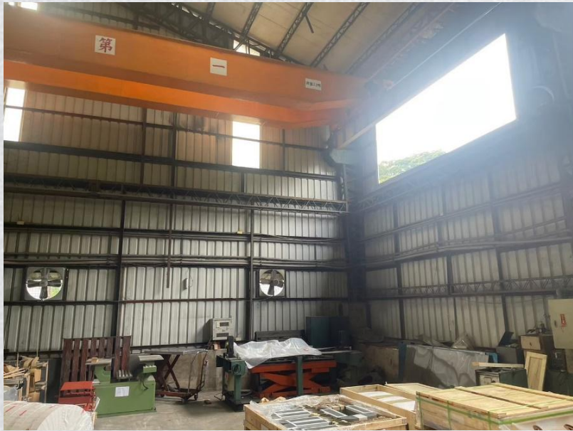
2.3cm Thick Composite Sound Insulation Panels (pre-construction)
