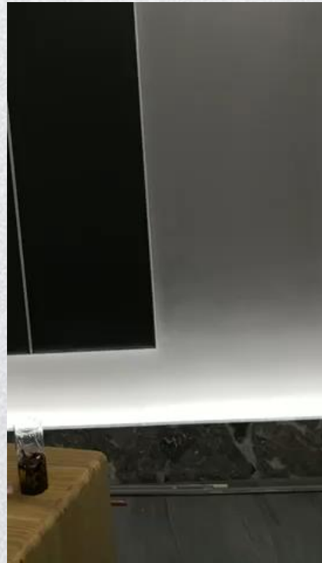
Reverberant Acoustic Panels (After Installation)
