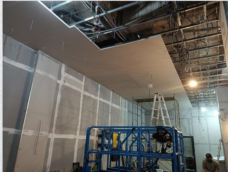
2.3cm Thick Composite Sound Insulation Panels (during construction)
