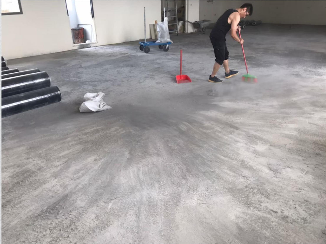
Polyester fiber vibration isolation blanket - Wet construction (pre-construction)
