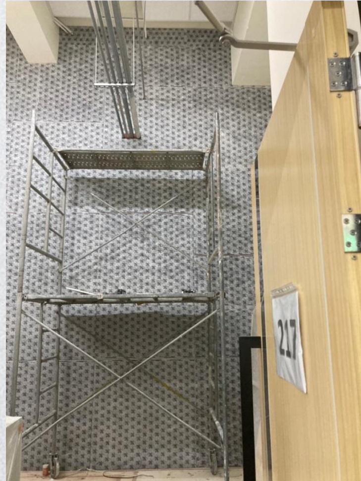
Sound Isolation blanket (during construction)
