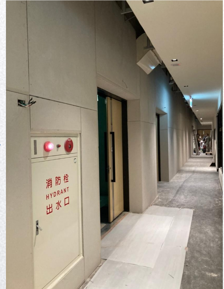
Sound Isolation blanket (after construction)
