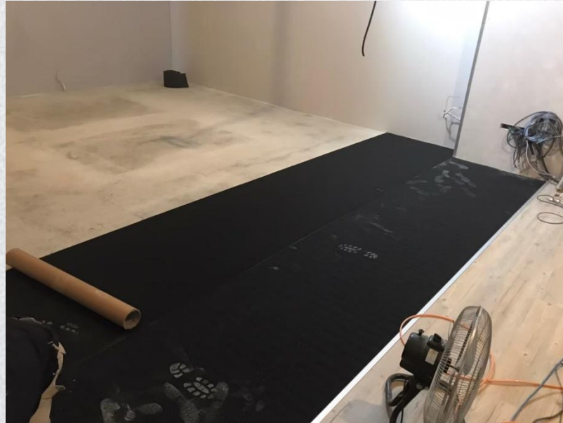
Rubber Anti-Vibration Pad (during construction)
