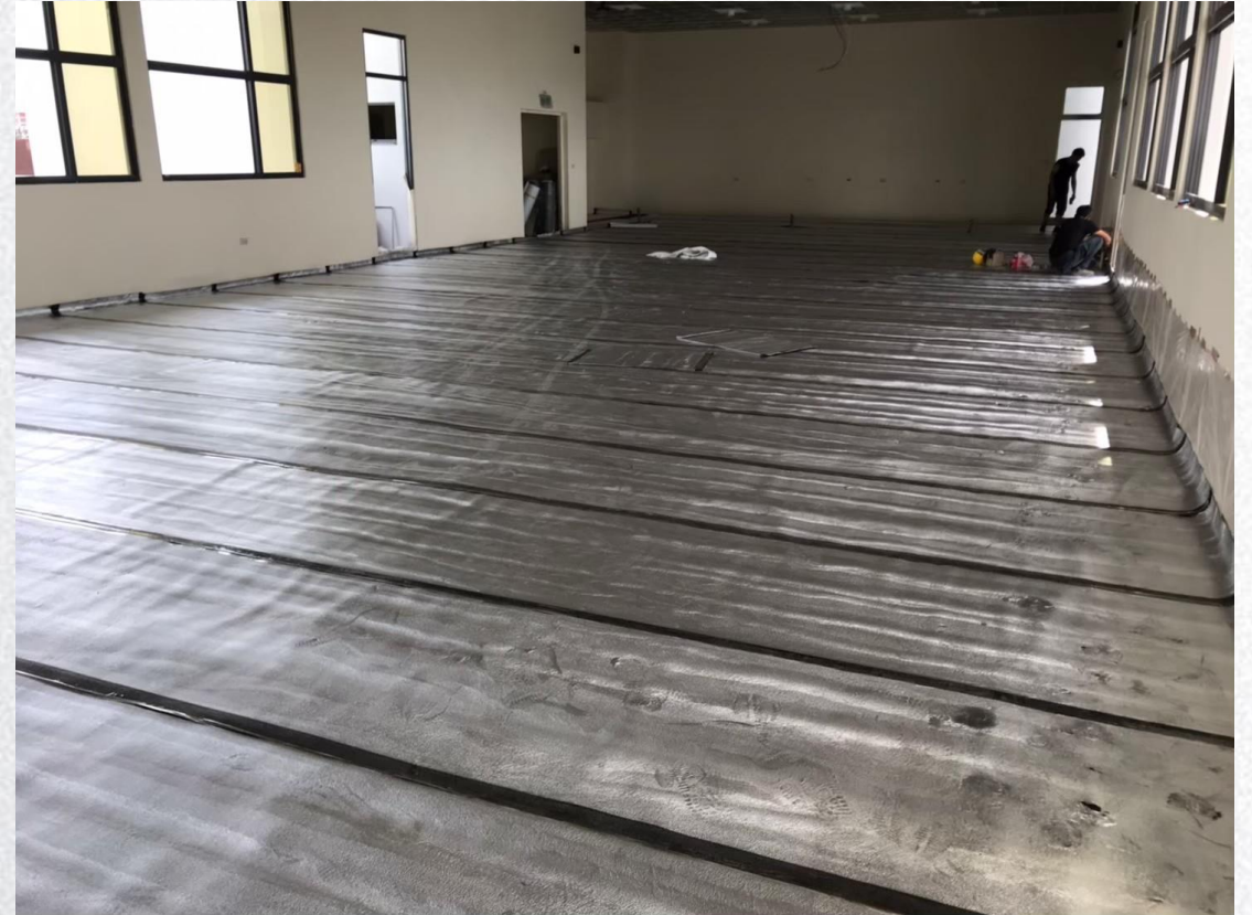
Polyester fiber vibration isolation blanket - Wet construction (after construction)
