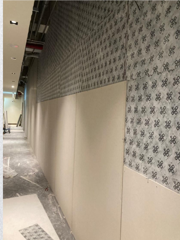
Sound Isolation blanket (during construction)
