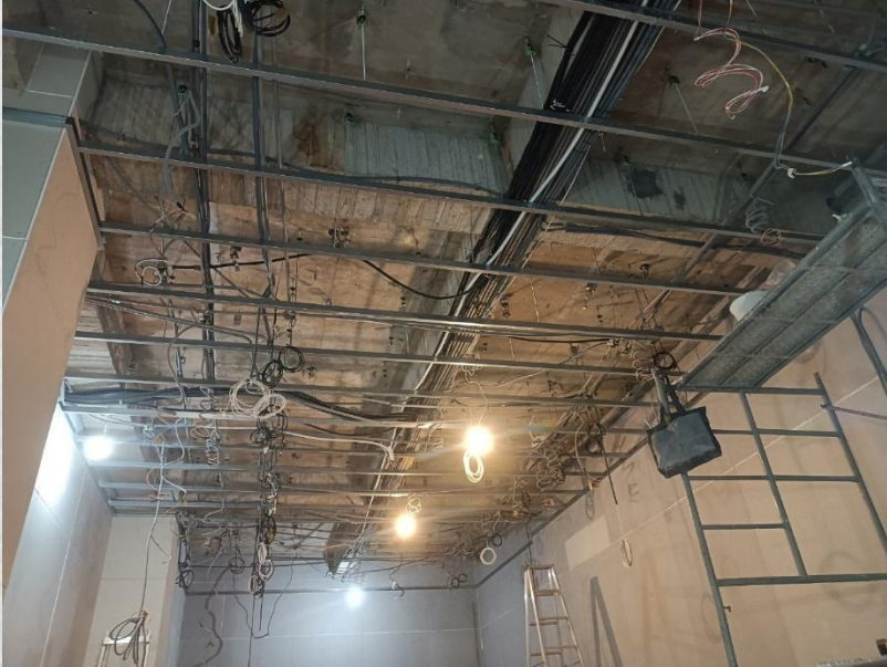
2.3cm Thick Complex Sound Insulation Panels (pre-construction)
